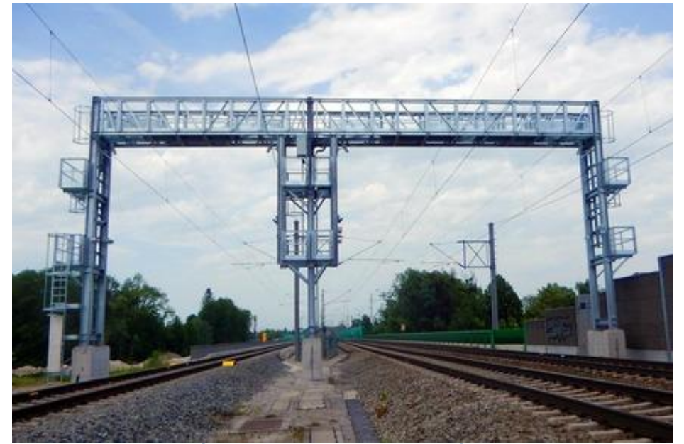
Checkpoint for supervision of rolling stock
